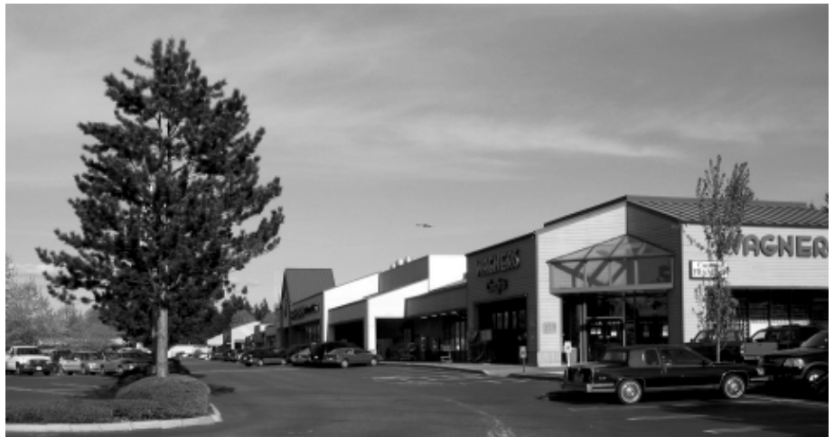
Covington Square in the newly incorporated city of Covington in King County. Strip malls are in many peoples' minds a particularly unattractive reminder of the need for growth management. The City of Covington recently lifted a growth moratorium which had been imposed due to lack of water. Their official motto is “Come visit us and see what develops here.”
